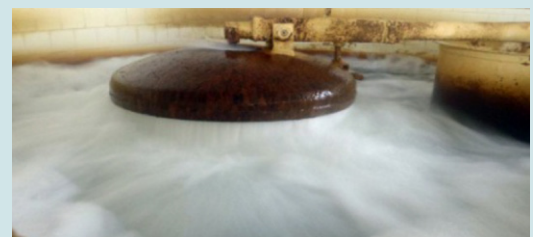
Figure 176 - Water pressure dissipation using a load breaker
